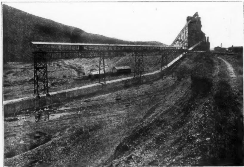
View of Wyoming Sand and Stone Company's Plant Showing Storage Distribution System and Tunnel for Reclaiming Material
